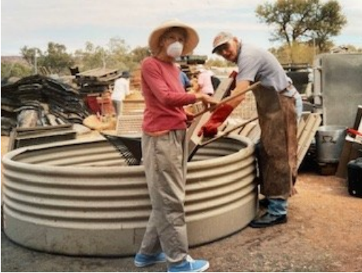
Wal working on the “Acid Bath” to clean off the dirt from the air conditioning louvres of St Philips College, Alice Springs.
