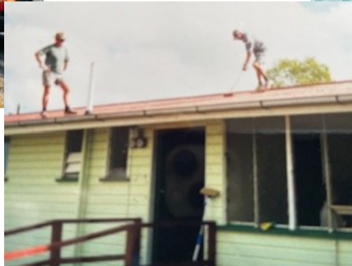
Scrubbing the roof
